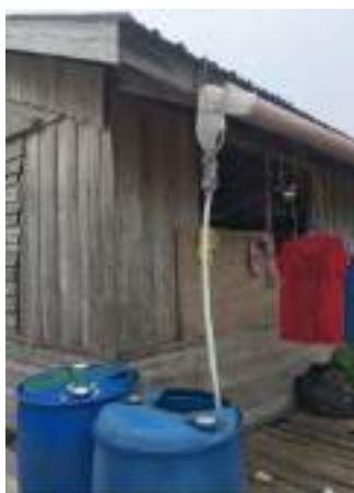
Rudimentary rainwater harvesting system for household use like laundry and cleaning.
